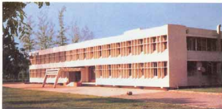
Manufacturing and Research & Development Centre, Navi Mumbai
